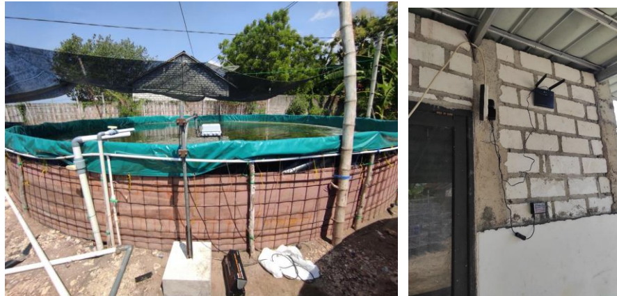
FIGURE 6. Node and master station installation
